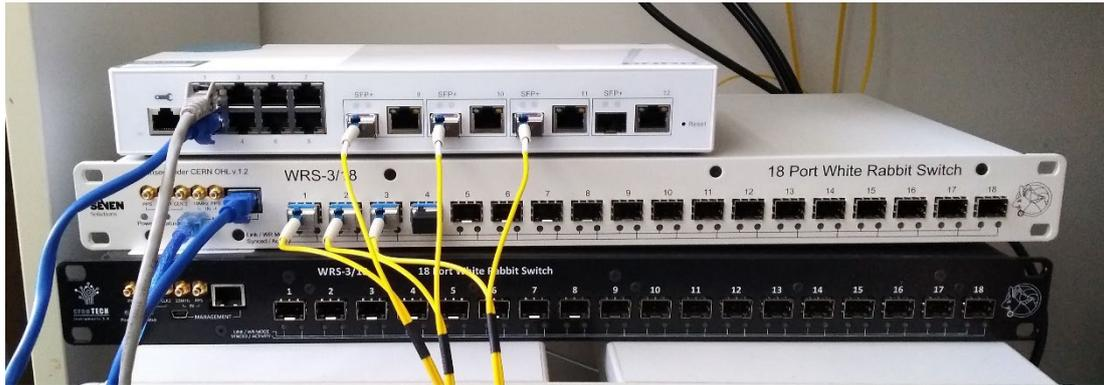
**Figure 2-16. Top to bottom: a) 1/10 Gb Ethernet switch for communication with the SDRs, b) and c) WhiteRabbit switch for precise timing**
